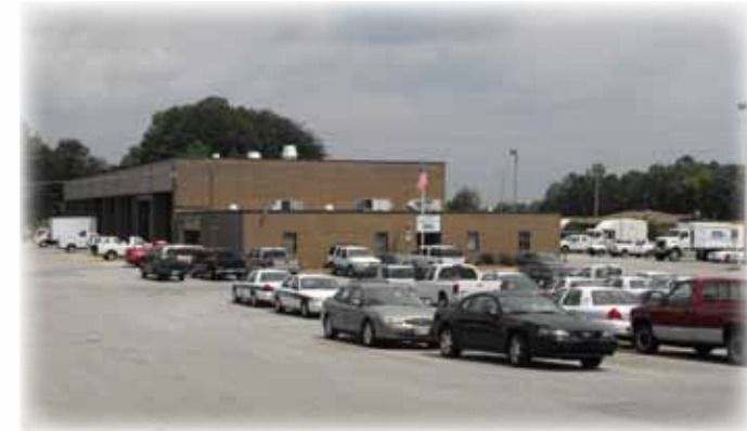
High Point Fleet Services building and grounds
