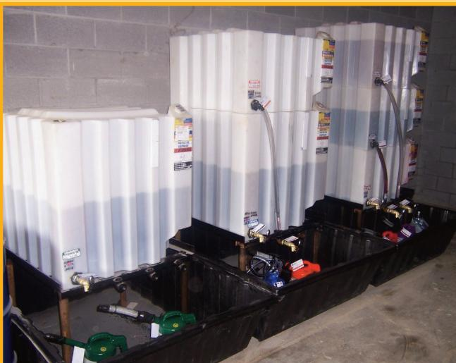
Lubricant storage room after the implementation of an RCM program – note the clear labeling and colour-coded Oil Safe containers as well as Tote-A-Lube storage
