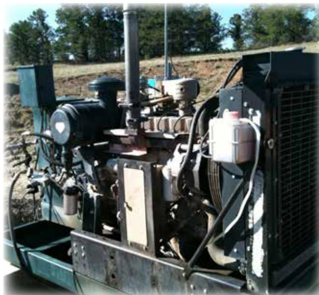
Cummins natural gas engine powered by coal bed methane
